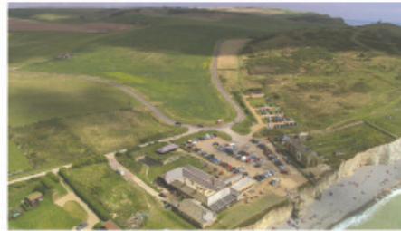
At Birling Gap the receding cliffs threaten the houses and hotel.
